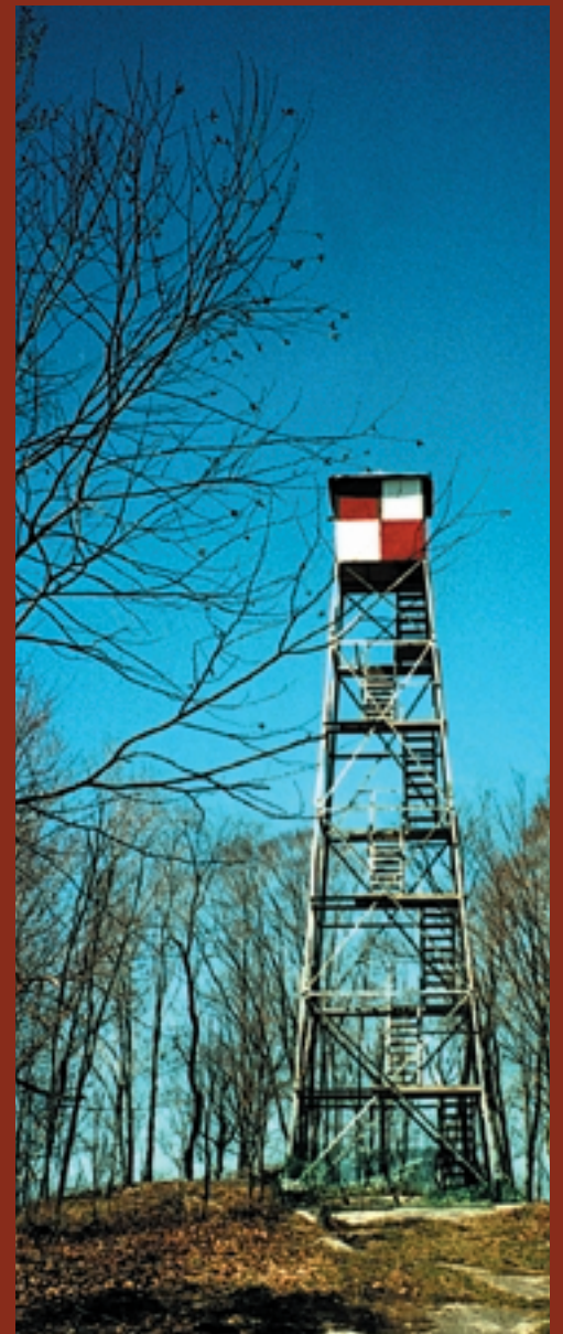
The Tooley Pond Mountain fire tower in its new home at the Ranger School.
