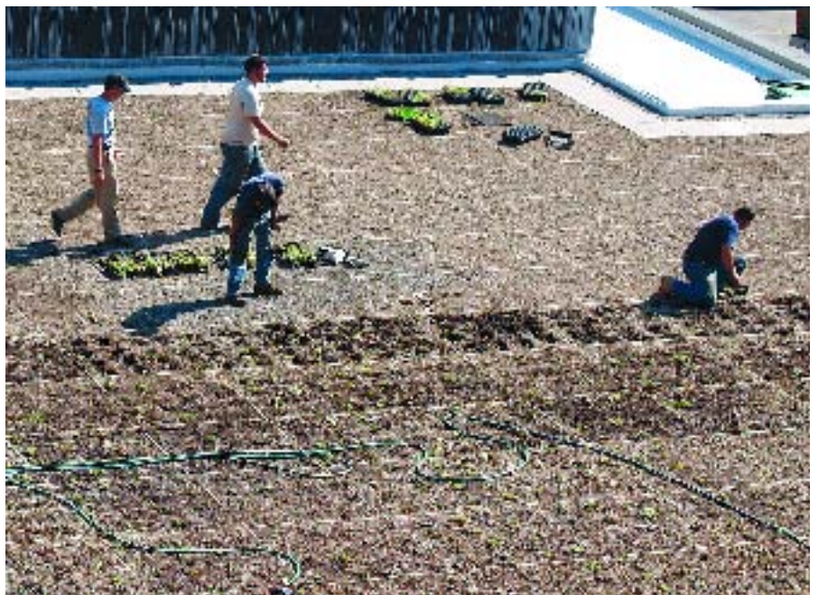
Workers install the green roof on Walters Hall.
