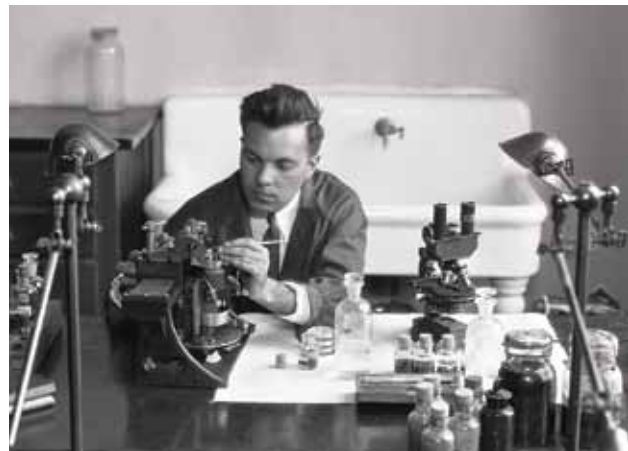
Student Cy Williams cuts sections of wood to 25/1000 of an inch in thickness as part of his course work in wood technology. Williams would then prepare the samples for use with a microscope at high and low magnifications; circa 1940.
